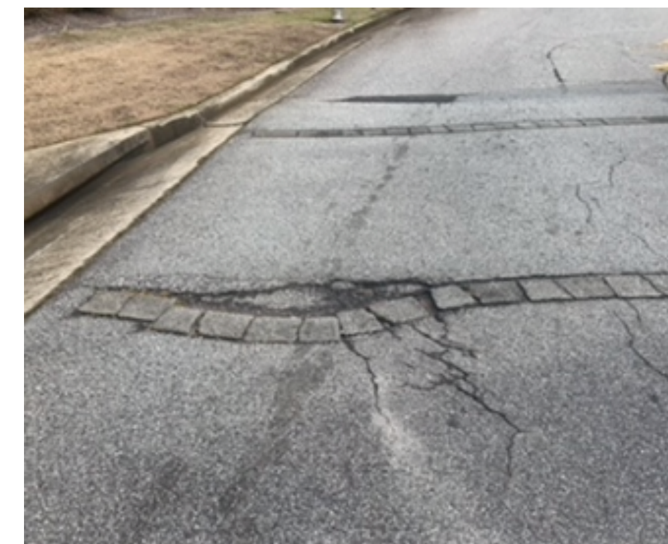
Speed Bump Repair
